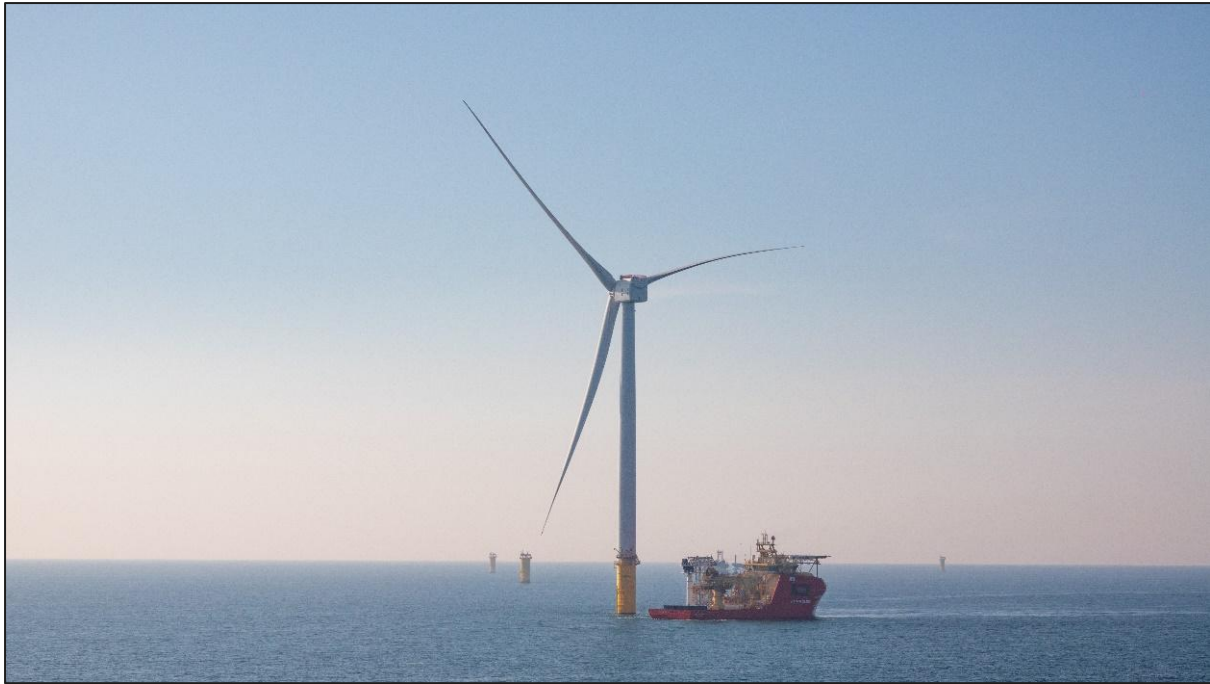
Figure 4.24: Installed offshore WTG with Monopile and TP installations in background (Photo courtesy of Dogger Bank Windfarm)
