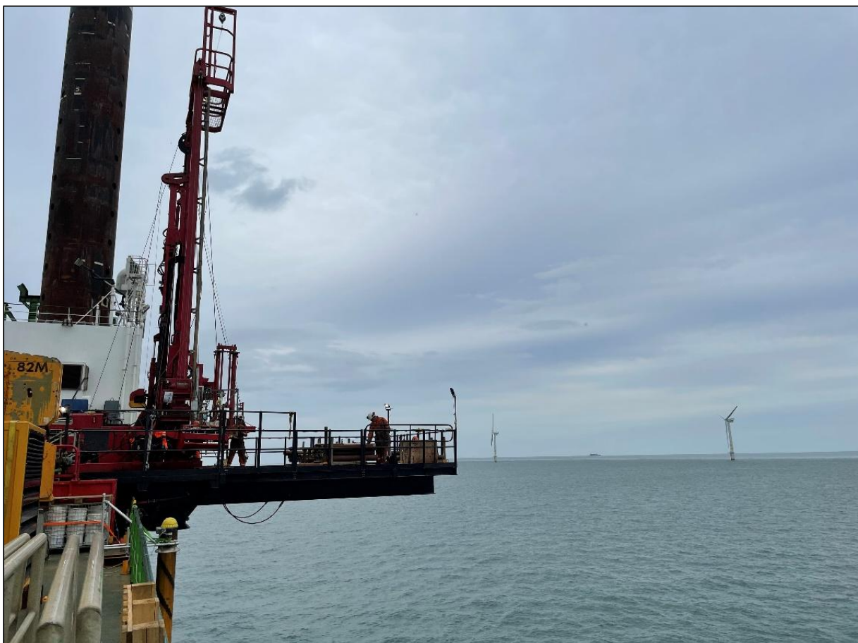
Figure 4.19: Borehole drilling rig at Arklow Bank
