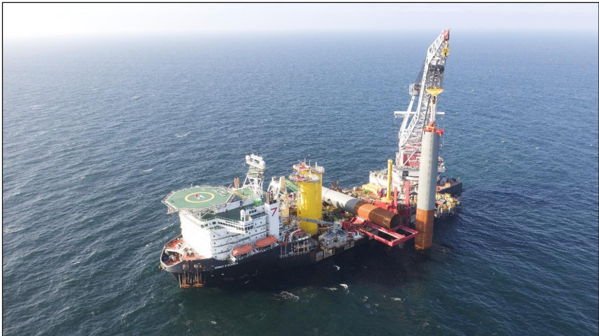
Figure 4.22: Monopile Installation (Photo courtesy of Dogger Bank Windfarm)
