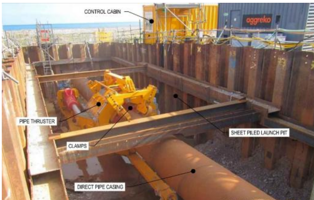
Figure 4.26: Direct Pipe Installation
