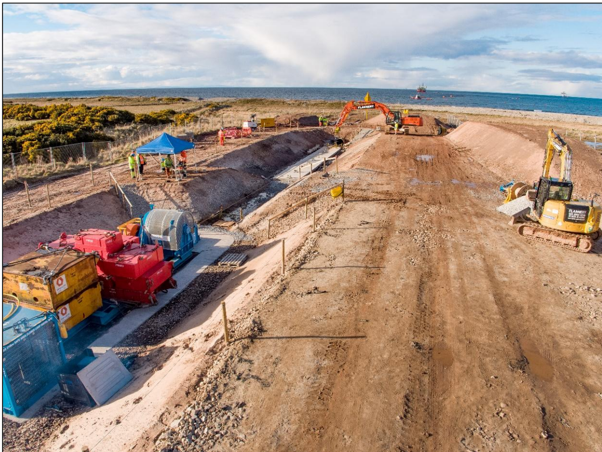
Figure 4.27: Offshore cable pull operation (Photo courtesy of Beatrice OWF)
