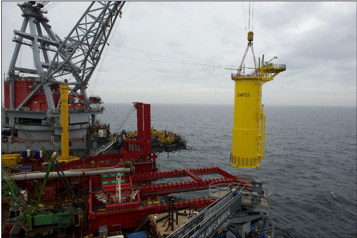
Figure 4.23: Offshore TP installation (Photo courtesy of Dogger Bank Windfarm)
