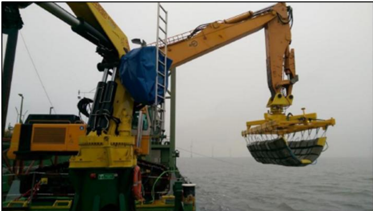
Figure 4.16: Concrete mattressing
