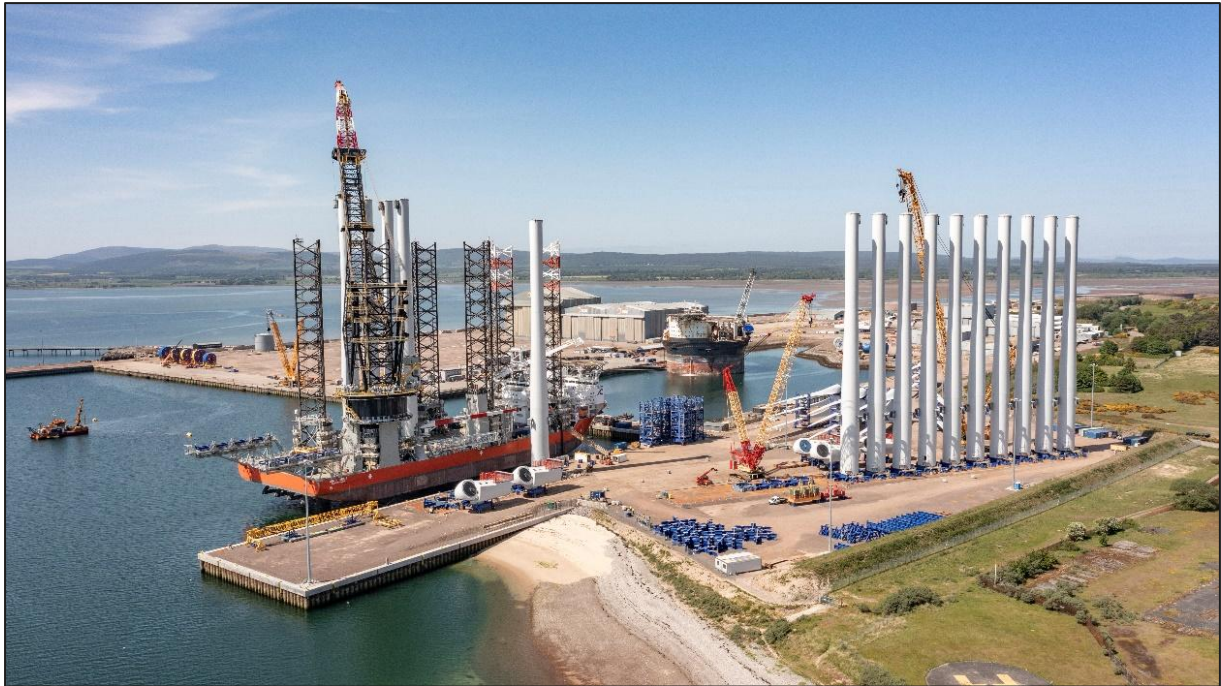
Figure 4.29: Construction port at Nigg (Photo courtesy of Seagreen OWF)
